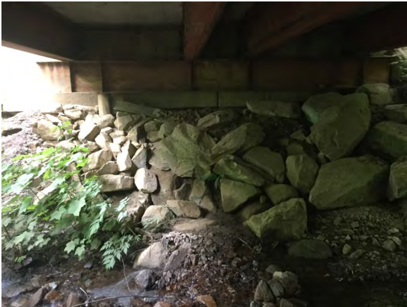
Right Bank Abutment when facing downstream
