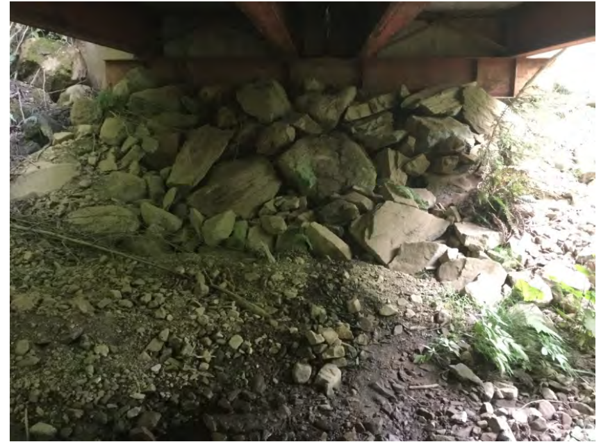
Left Bank Abutment when facing downstream
